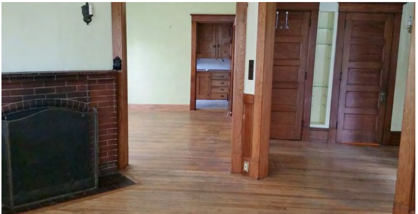
Figure 13. Interior of building located at 66 Barnes Ave. Original features visible with minor modifications.
