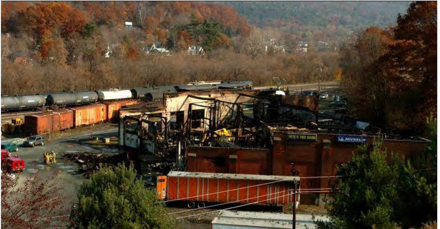
Figure 16. Image depicting remains of Roundhouse in Hartford after tire fire damaged most of interior and part of exterior.
