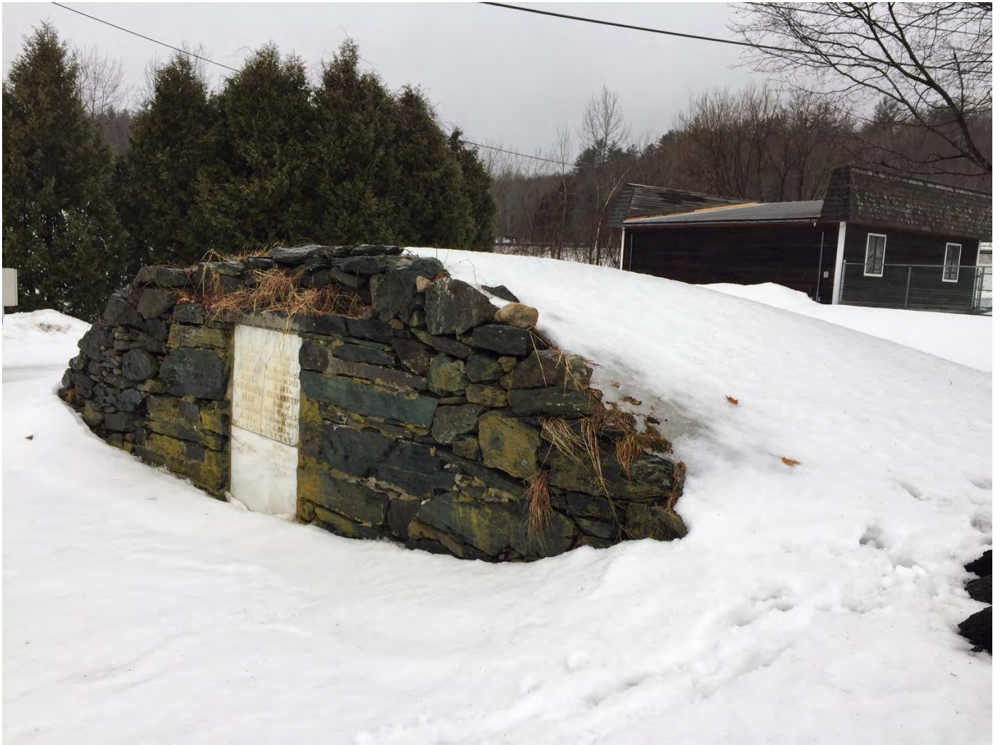
Figure 9. Wright's Tomb exemplifies a half-mound burial with tightly laid stones and marble work at its front: a classic burial vault type as listed in the Historic Context of Burial Vaults for the State of Vermont.
